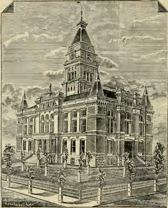
MONTGOMERY COUNTY COURT HOUSE.
